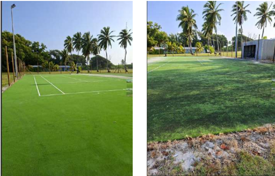
Figure 2: Cleaning of tennis court surface continued in August 2026. Half the court has now been washed. This will continue in September.
