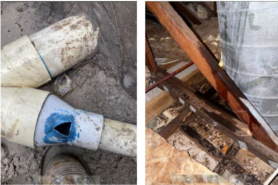
Figure 5: Plumbing repairs and replacement of hot water units to houses on Home Island.
