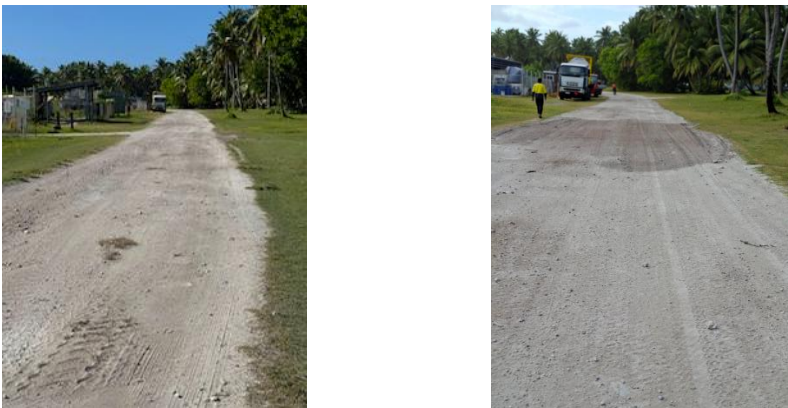
Figure 7: Pothole repairs on Home Island.
