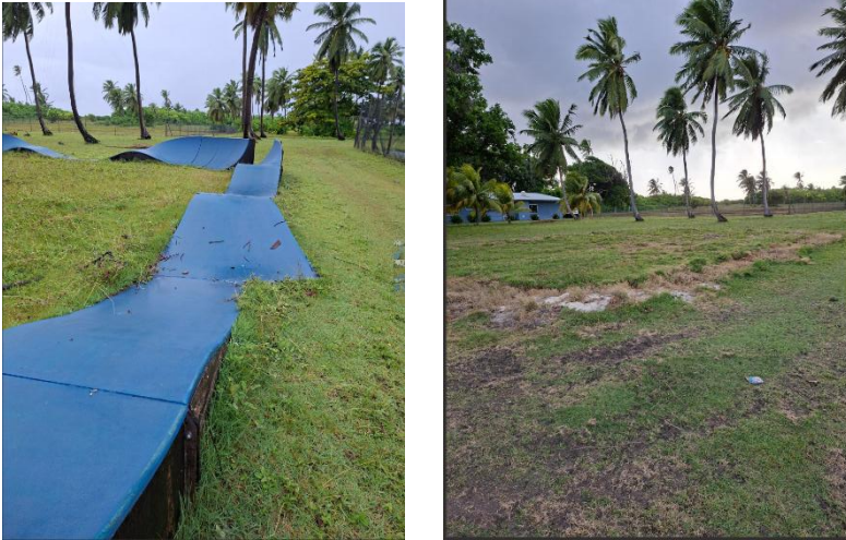
Figure 1: Removal of the pump track.
