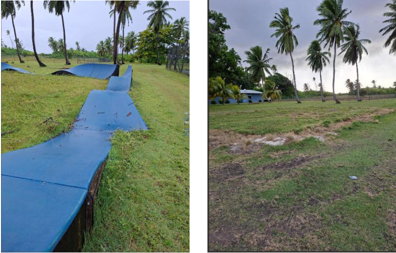
Figure 1: Removal of the pump track.
