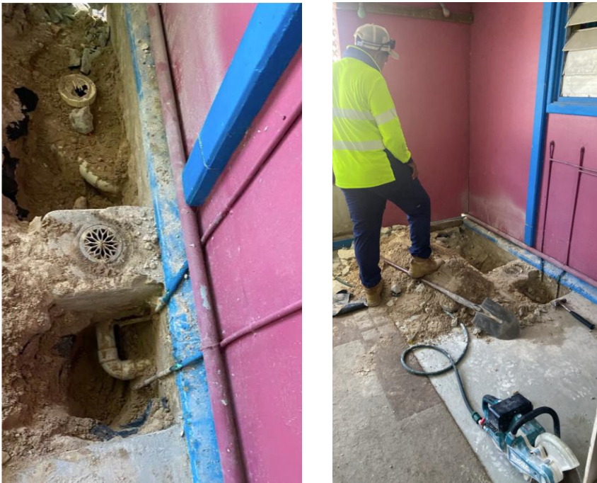
Figure 5: Plumbing repairs to a house on Home Island.
