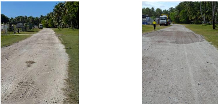
Figure 7: Pothole repairs on Home Island.
