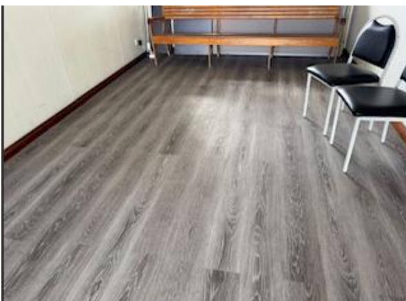
Figure 6: New flooring was installed in the Community Resource Centre on Home Island
