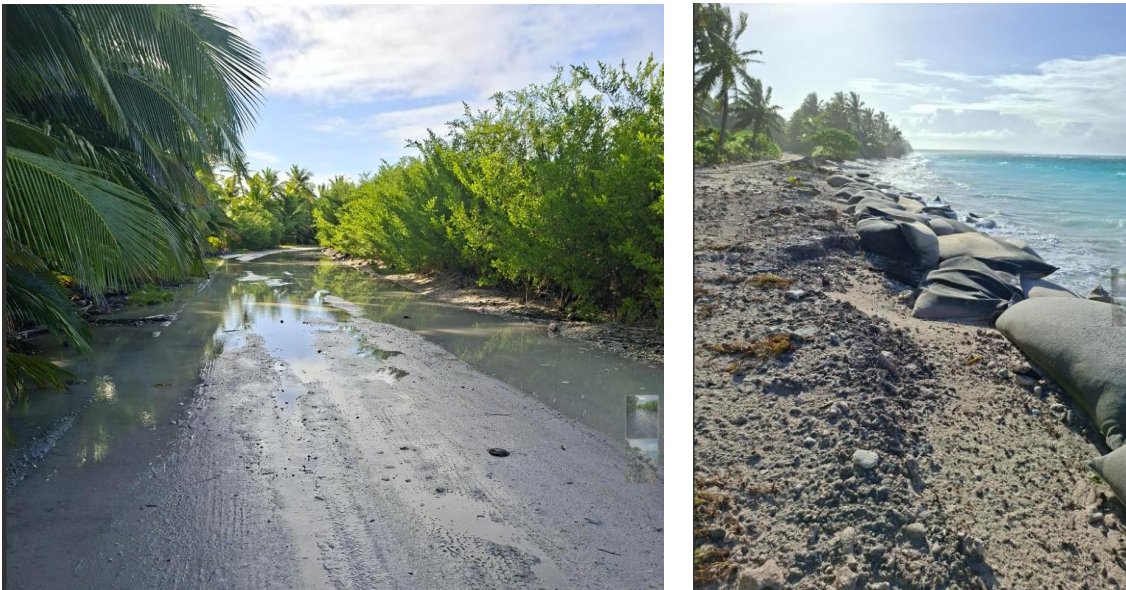
Figure 6: Tidal flooding in August delayed minor grading works on South Rd and impacted on transfer of grader, roller and excavator for the road program on Home Island.
